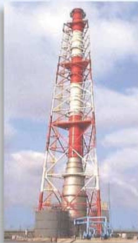
AirPol Absorber for a 60 MW Coal Fired Co-Generation Plant
