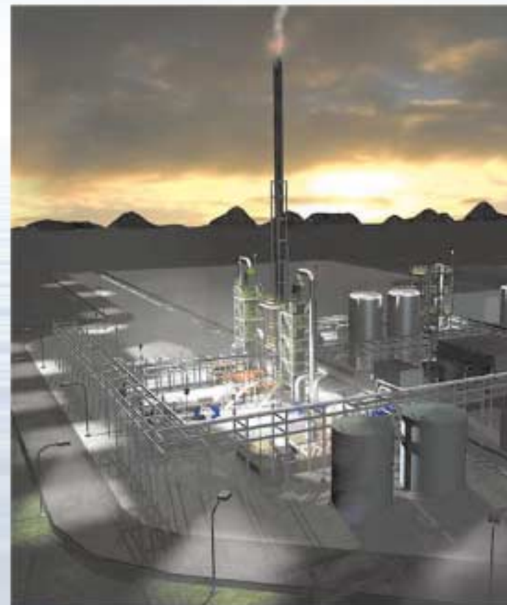
AirPol air pollution control system consisting of two quench-absorber trains for a hazardous waste incinerator plant.
